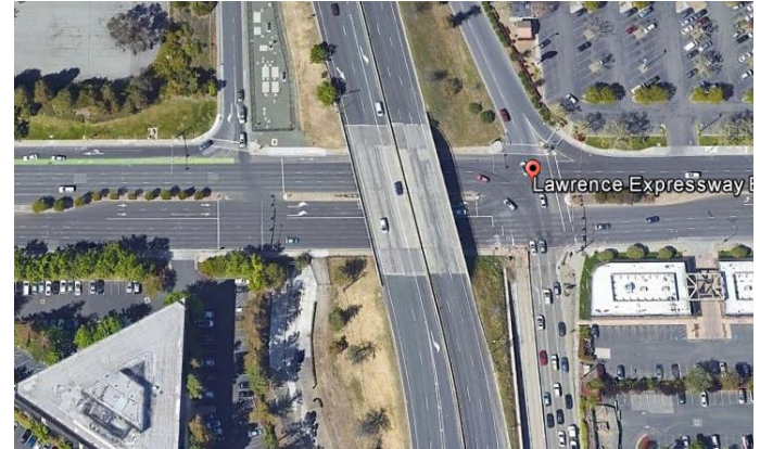
Lawrence Expressway ramp improvements
